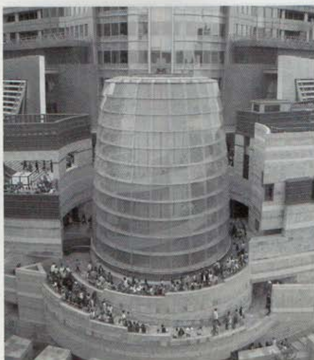
写真4 昼建物外観 Photo 4 Day time exterior view
