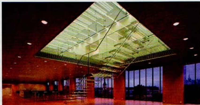
第3章-3 ガラス階段 (35頁) ©Adam Mark Structural Glass Staircase in Denmark
