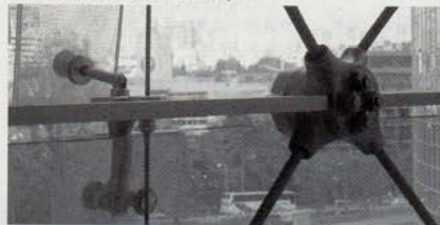
写真8 圧縮リングと金物2 Photo 8 Compression ring and stainless fittings 2
