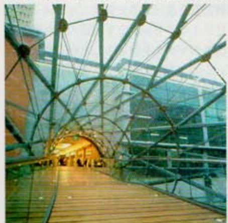
第3章-3 内観 (36頁) ©Barnard, O'Sullivan Street Footbridge in Manchester
